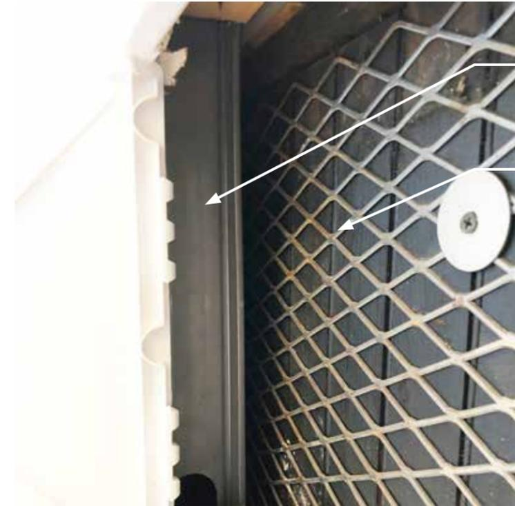
NEW STEEL STUD CONSTRUCTION (NOT ORIGINAL)
