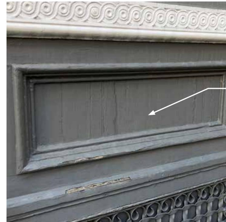
PLYWOOD BEADBOARD AND TRIM ATTACHED TO NEW STEEL STUD (NOT ORIGINAL)
